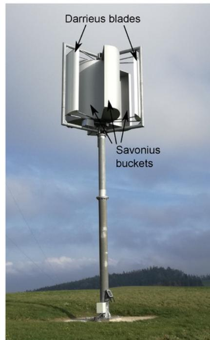
Figure 7. H-Darrieus turbine with hybrid rotor configuration [78].
